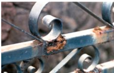
Fig-2 Corrosion of Railings
