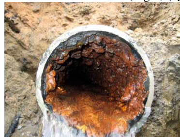
Fig-1: Rusting in a drainage water pipeline
